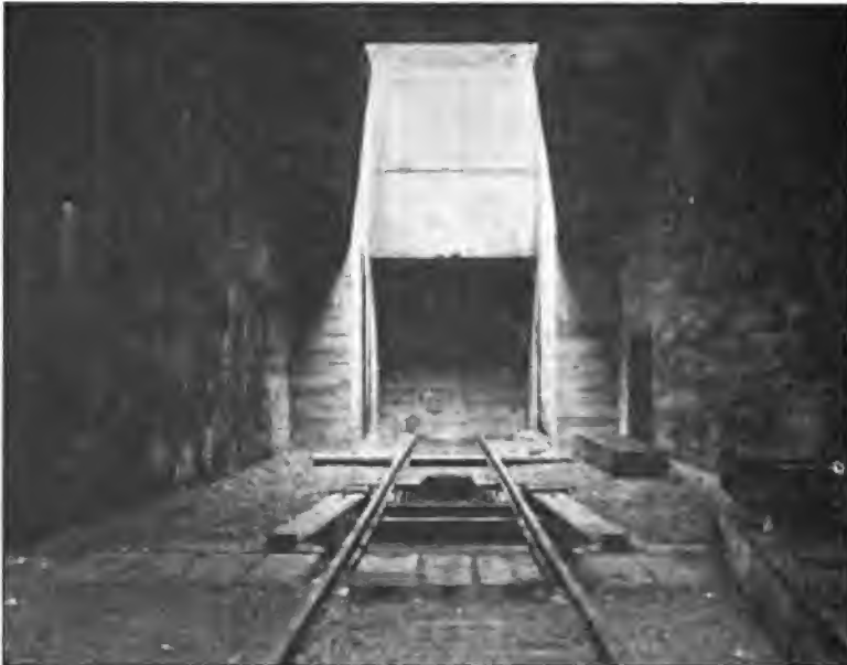
INTERIOR OF CONCRETE EMPLACEMENT FOR 340-MM. FRENCH GUN (CON- STRUCTED BY AMERICANS).
